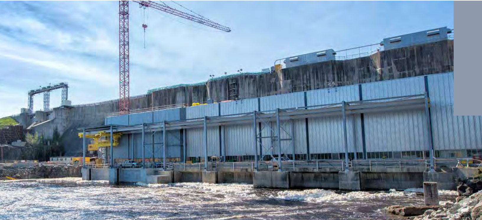
Lower Mattagami, Kipling GS construction
