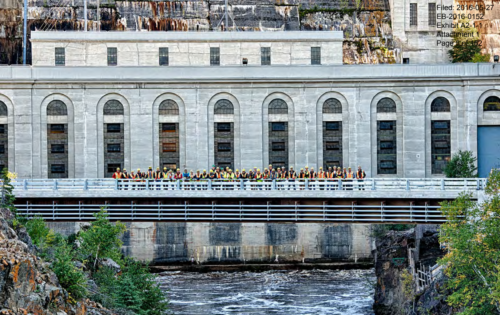
The old Smoky Falls generating station, Lower Mattagami Project.
